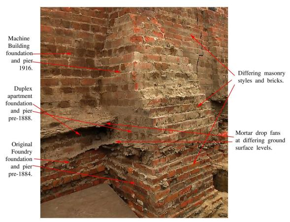
Figure 9 Buttress and structure of the eastern foundation wall.°
