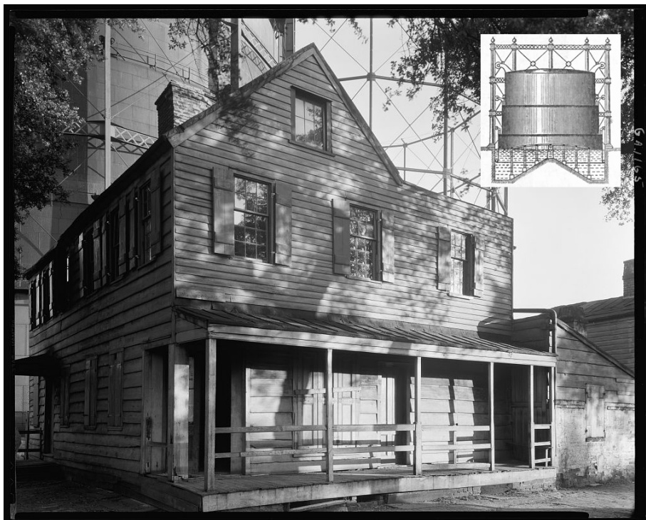
Figure 6. Trustees Garden Gasometer cylinders and frames were visible in the background of this Library of Congress photo from 1939. The building later became the Pirates House Restaurant. The upper right inset shows the telescoping process of Gasometer tanks.
